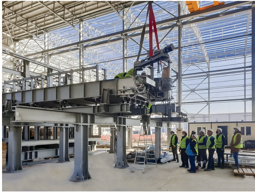
On site team training at new furnace build, Turkey 2021
